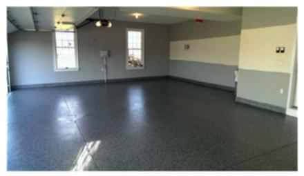
• Tool Joints – Are filled with an epoxy paste. The joints later appear as decorative lines in the floor finish.
